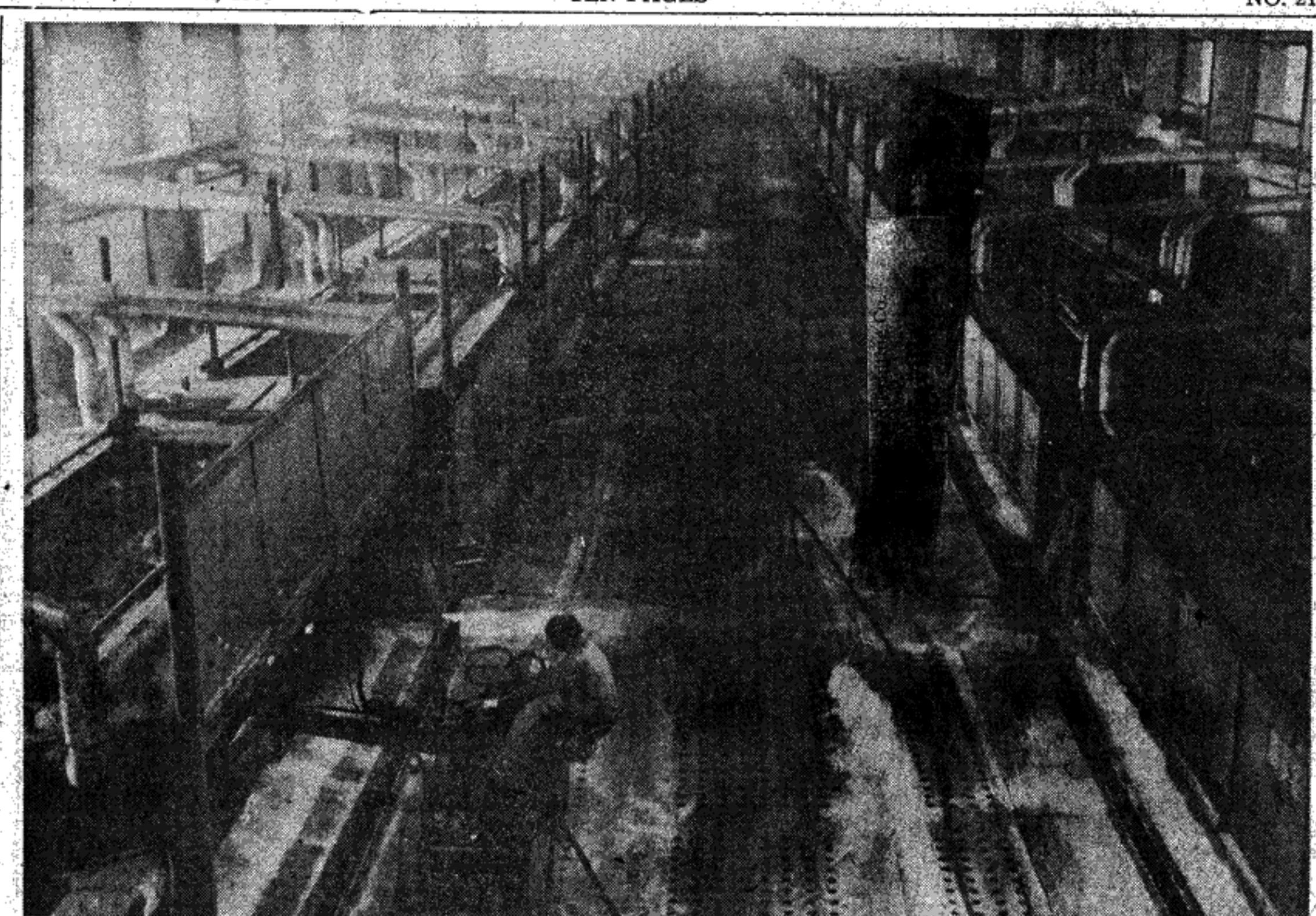
BIGGER THAN FOOTBALL FIELD—More than three times as long as a football field is this potroom at the Reynolds Metals Company Listerhill Reduction Plant. There are nine such potrooms in the new plant here and five smaller ones in the older but since modernized plant. Each of the 56 pots in this room can produce 1225 pounds
