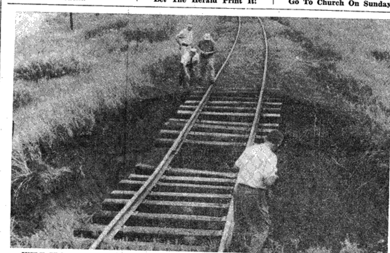
WIDE SPOT IN THE ROAD —No less than 11 railroad cars were pulled by a locomotive across this natural trestle in Kingdom City, Mo. The road bed fell into an abandoned quarry, leaving a hole 100 feet deep. Nobody knew what happened until after the train passed safely over the gap.
